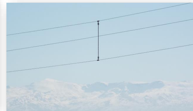
Installations in Southern Spain – 2017-2020 Network 15/36kV. Total separation distance between phases: 1.5m – 2.8m.
