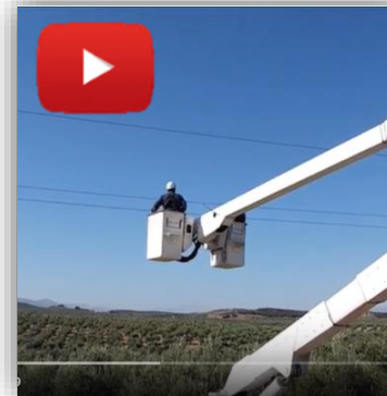
Installations in Southern Spain – 2017-2020 Network 15/36kV. Total separation distance between phases: 1.5m – 2.8m.
